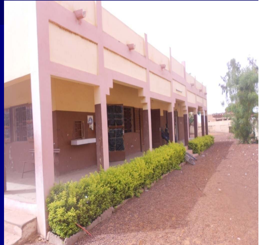
Dioro Health Center
